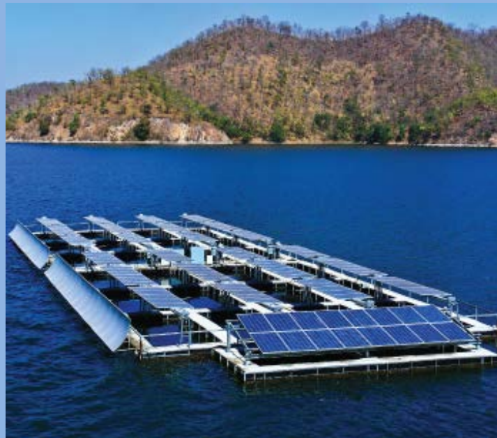
A solar and tidal energy farm in China
